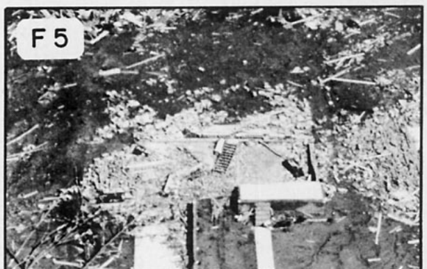
FIG. 8. Reference photographs of F2–F5 damage, which correspond to the F-scale damage specifications being used in rating U.S. tornadoes for producing and updating NSSFC and DAPPL tornado tapes.
